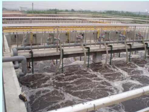
Submerged Membrane Bioreactor plant in Simona Tanning for water recovery
