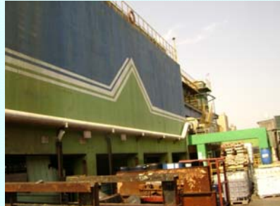
TANNERY EFFLUENT TREATMENT PLANT IN MULTI STORY LEVEL –
