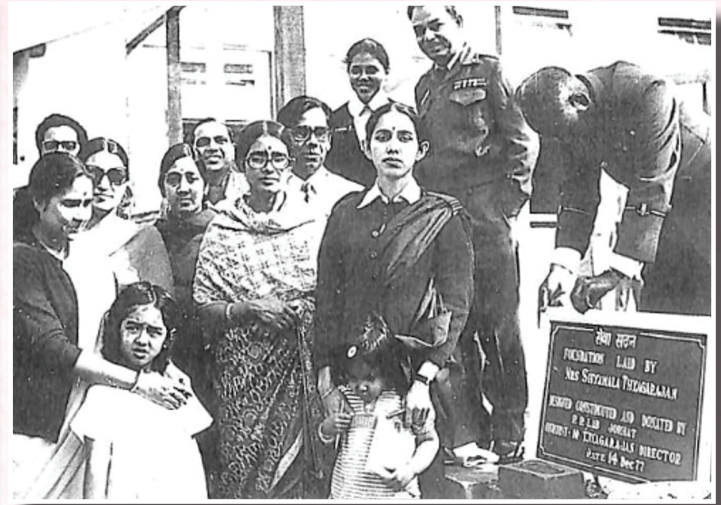
GT at proving on the ground: The foundation stone for low cost housing unit being laid at Jorhat with RRL Technology
